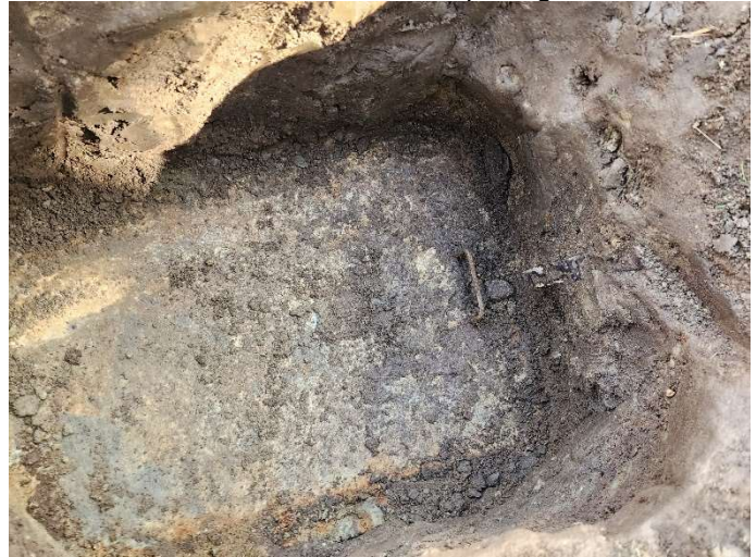
Picture of distribution box before opening
