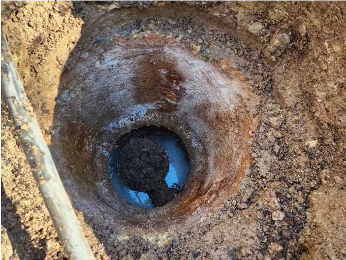
Picture of outlet after opening
