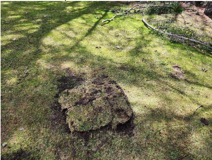
Picture of distribution box buried
