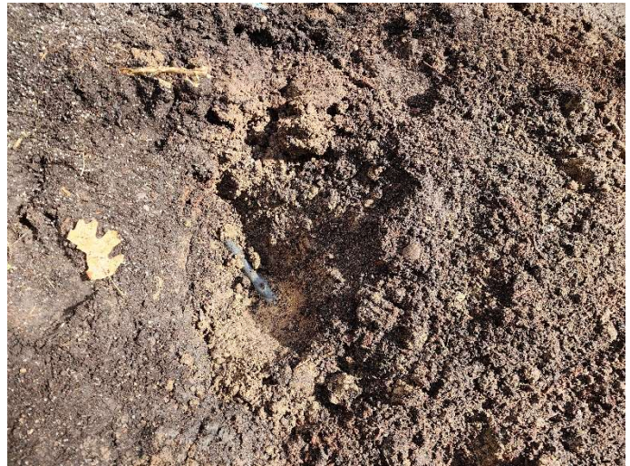
Picture of tank buried except irrigation line
