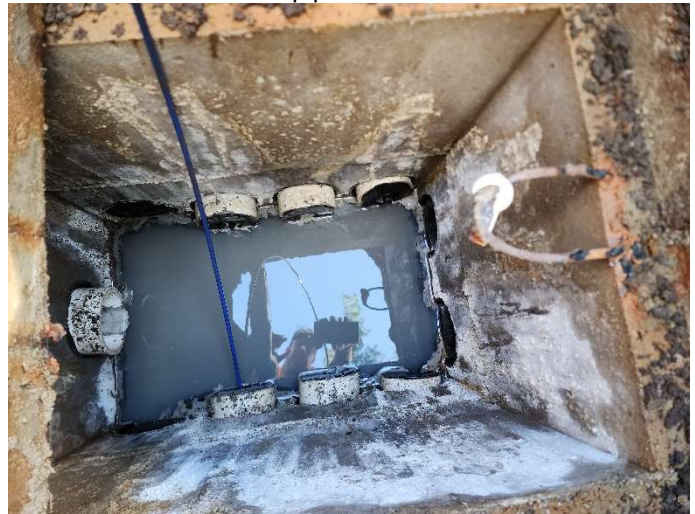
Picture of camera in third outlet pipe
