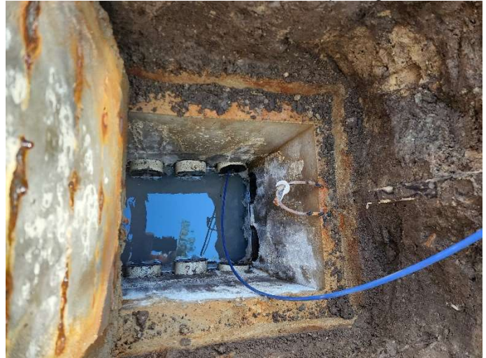
Picture of camera in first outlet pipe
